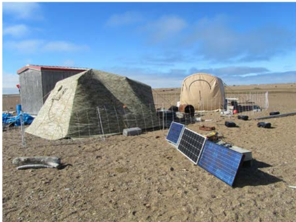
Solar panels for the radio station
