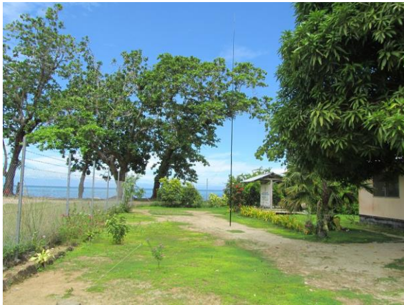
Antenna setup at the Provincial Guesthouse
