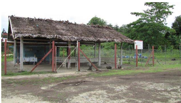
Airport Terminal Santa Cruz
