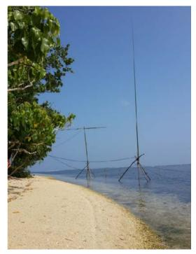
The next job is to attach the antenna to the mast of the bamboo plant and some branches of wood as a buffer so that the antenna can stand . This job is quite difficult because the ground is the sand and stones. Finally at 13.00 noon all antennas can stand perfectly.
