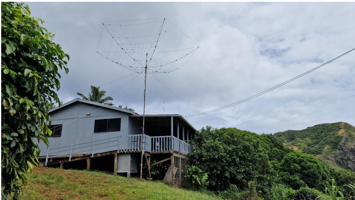
Figure 15 - The Hexbeam nicely attached to the veranda
