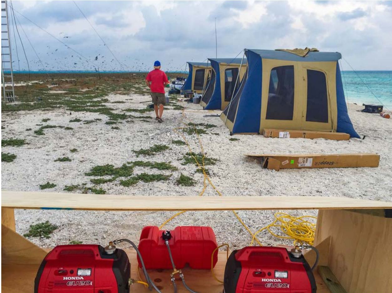
Figure 5 Main camp - Generator shelter located at the main camp.
