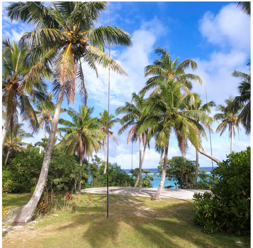
Photo 19 – 40m 4-Square installed among the Coconut trees
