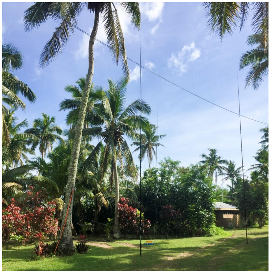
Photo 20 – 30m 4-Square installed across the drive-way (telephone lines running through the middle)
