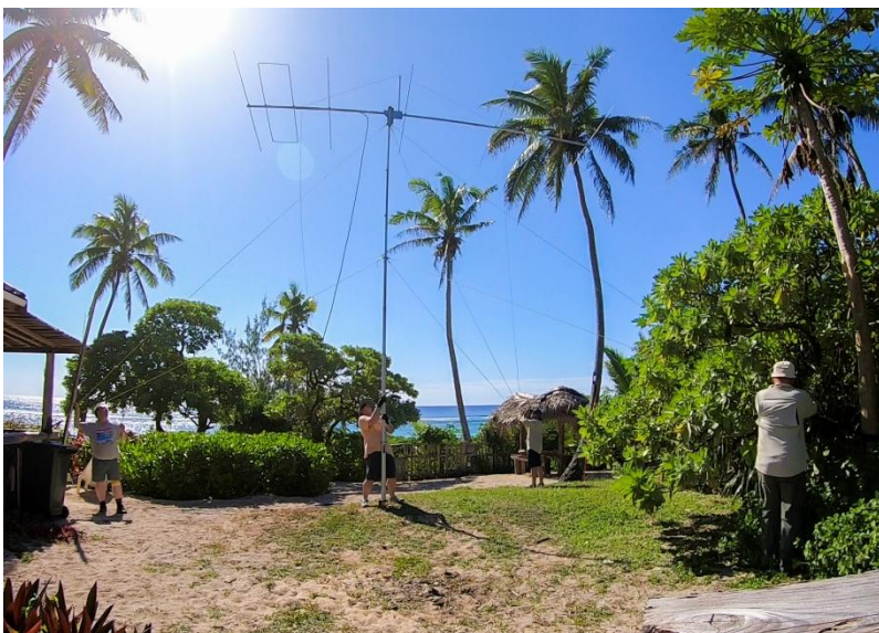
Photo 16 – Erecting the 6m beam – a team effort
