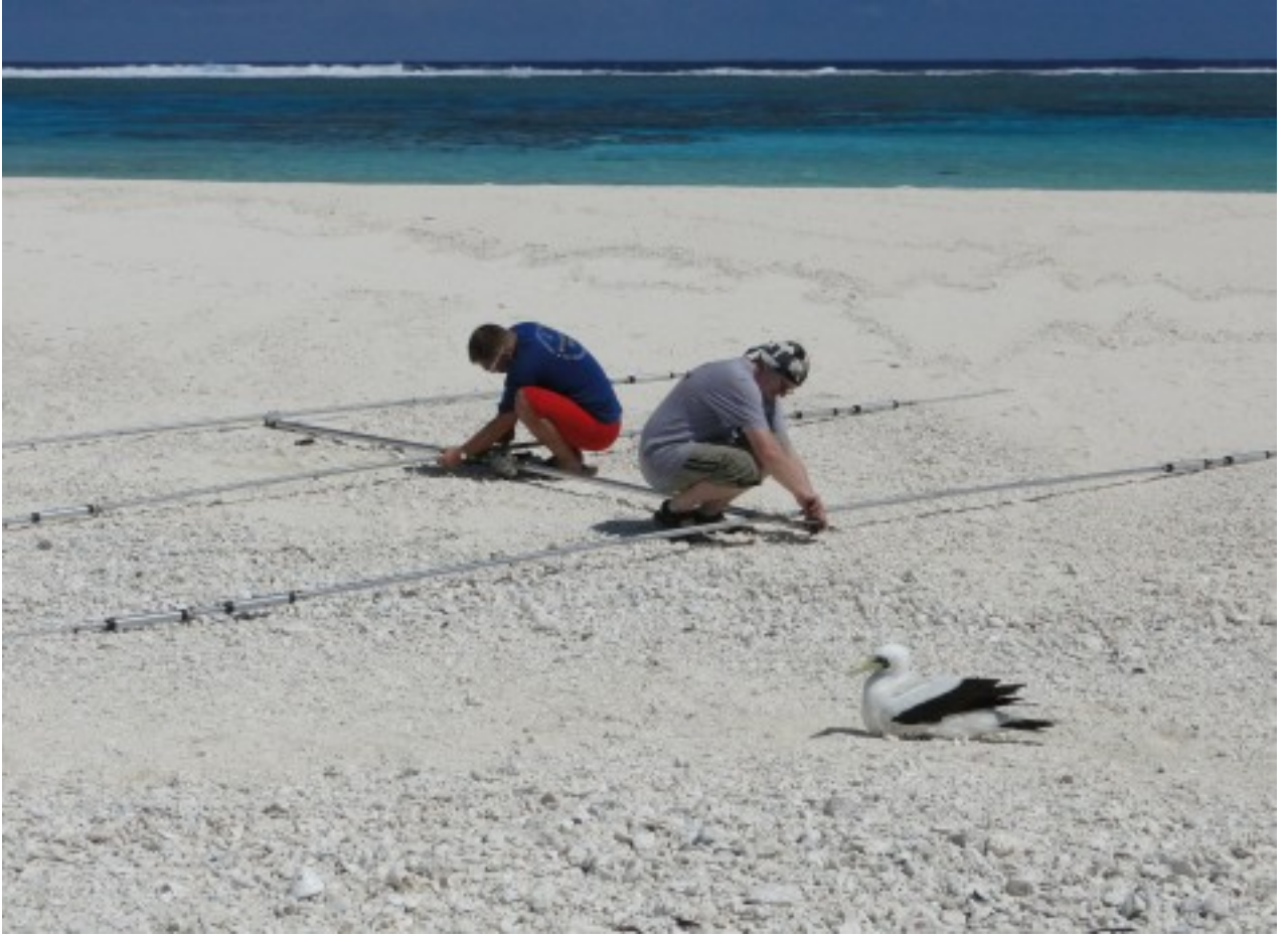
RZ3FW and UA4HOX assemble a yagi under the watchful eye of a nesting masked booby.
