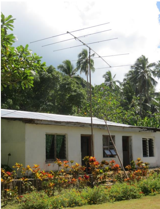
Left: The Cushcraft A50-5S 50 MHz yagi on its 6m galvanized pipe mast. Right: The horrific condition of the box in which the Spiderbeam had been stored!
